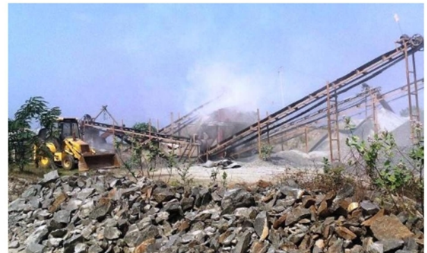
Stone- Quarrying activities
